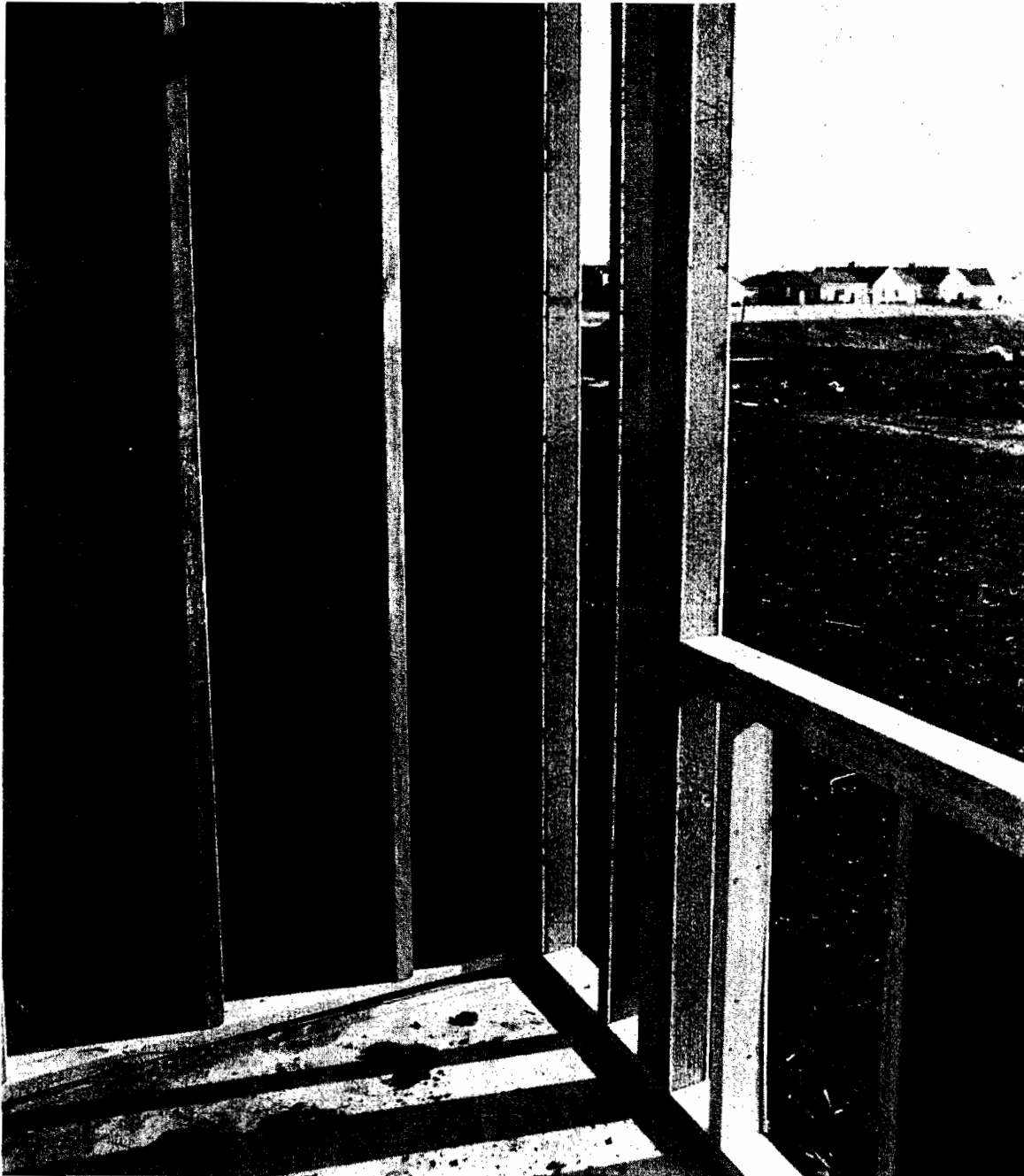
Figure 23.--COM-PLY studs used for window cripples.
