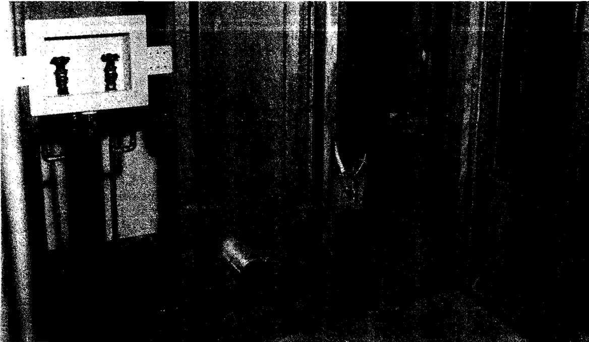
Figure 28.--COM-PLY studs were used to frame the interior partitions of NASA's Project TECH house. Large holes were drilled through the cores of the studs to accommodate plumbing.
