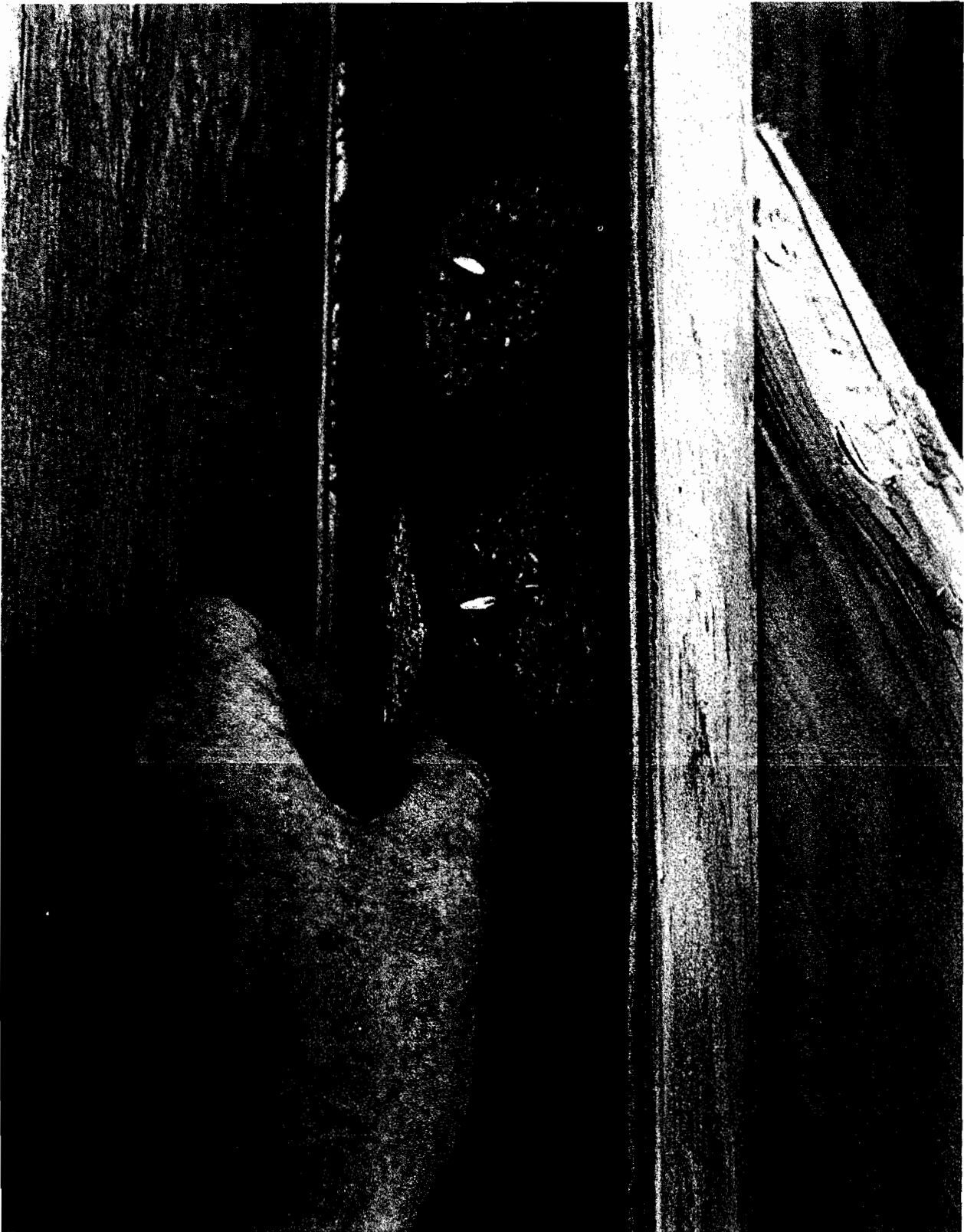
Figure 7.--Spalling occasionally occurred when nails penetrated the particleboard of COM-PLY studs.
