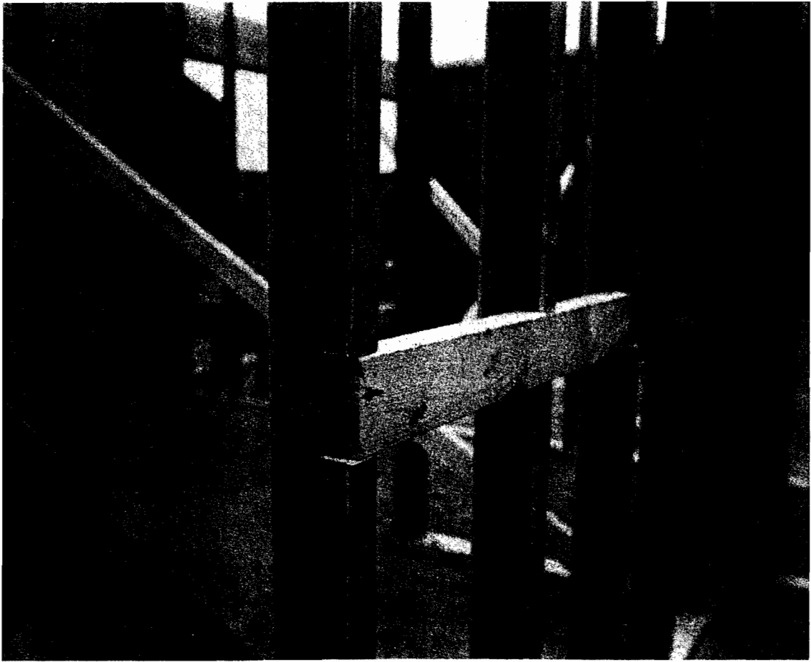
Figure 10.--The builder notched COM-PLY studs to install kitchen cabinets.
