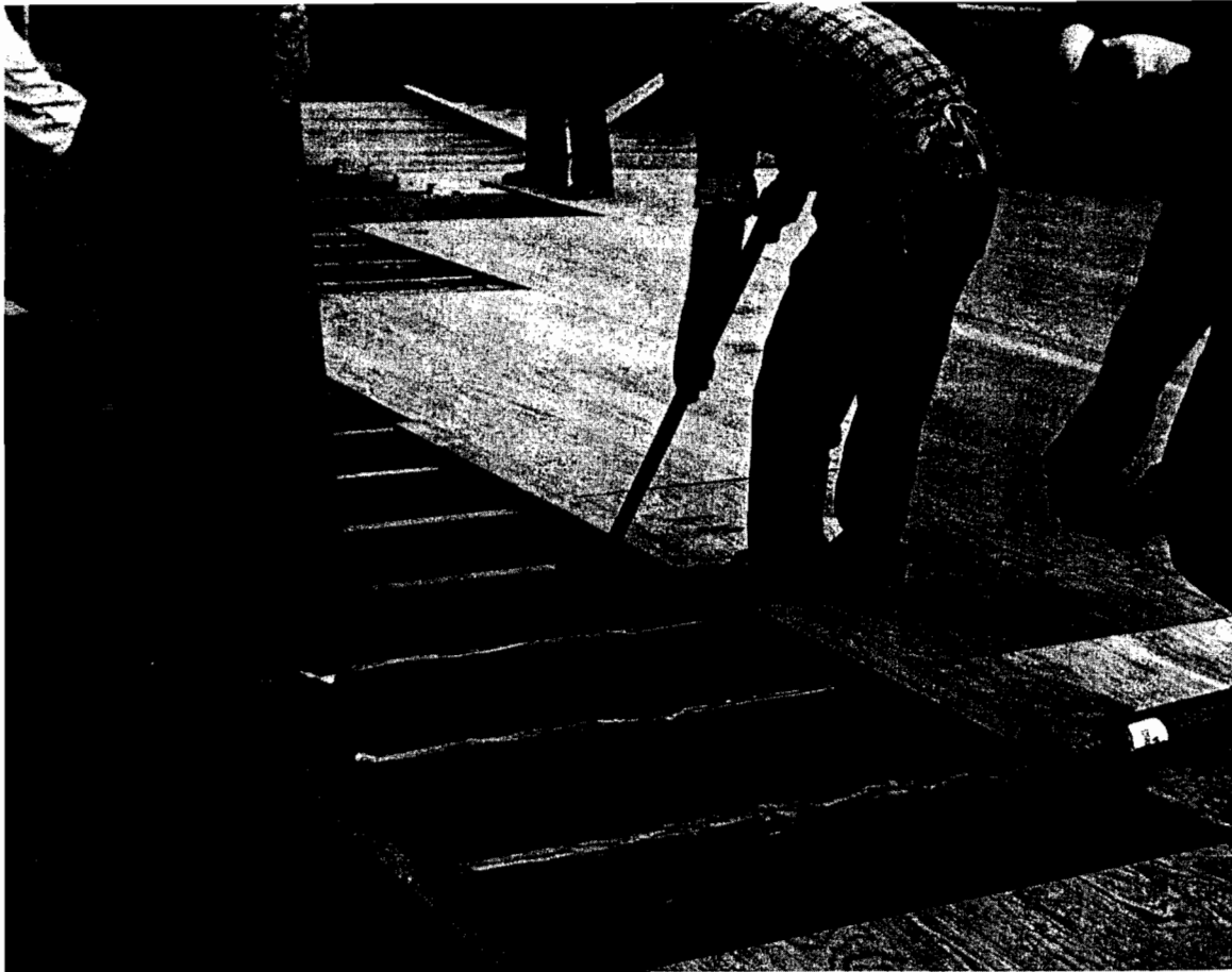
Figure 15.--Laying the composite floor panels. Note the tongue-and-groove joints.
