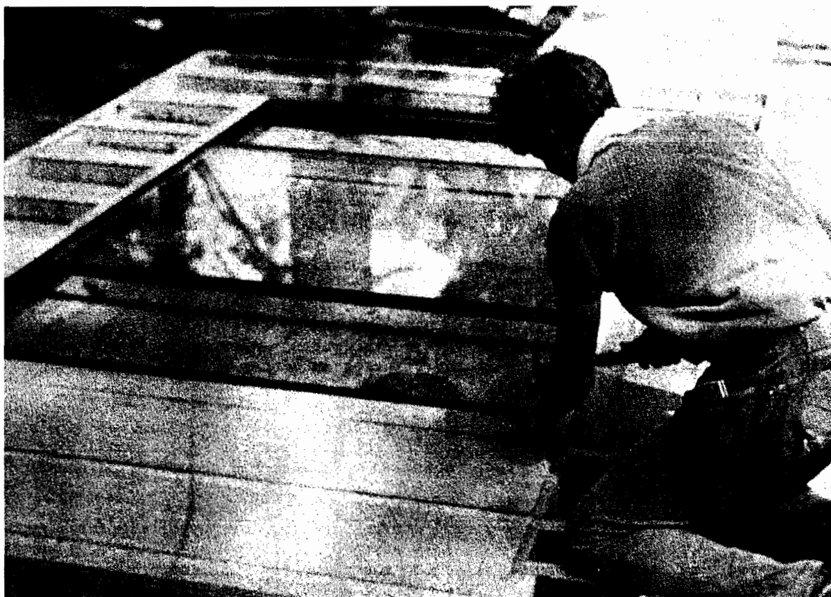
Figure 18.--Attaching the siding panels to the framing.
